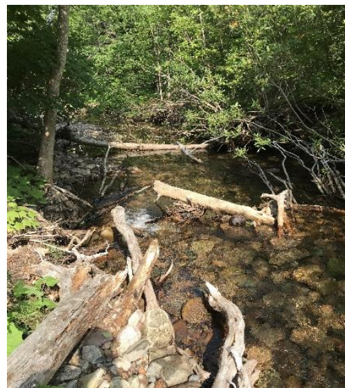
3b – New channel with trees in substrate
