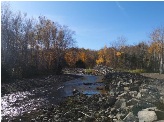
2b –Armour stone and rock berm above Alfred’s cabin (2020/1)
