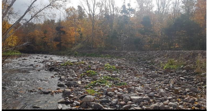
2b –Rock berm after being lowered in 2020 as part of restoration work
