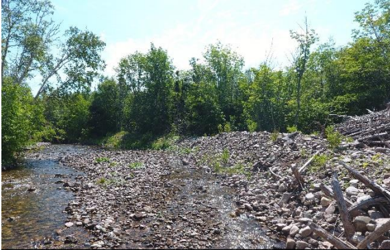
2b –Rock berm above Alfred’s cabin before restoration project (2020)
