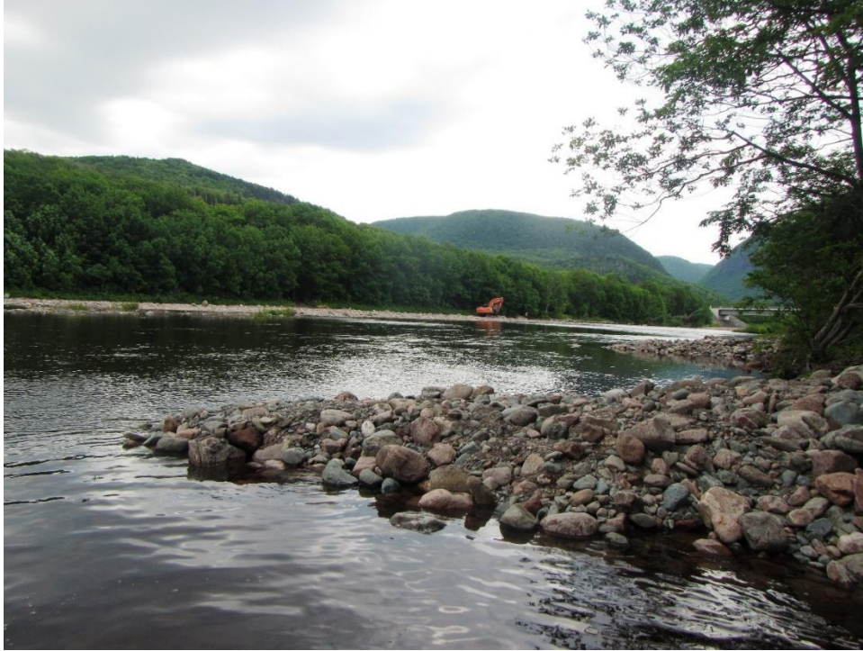
Site 5a. Restoration structures during installation, completed structure in the foreground
