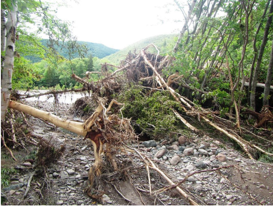
Figure 2a. Location at Robert Brook Site where access road damaged riverbank
