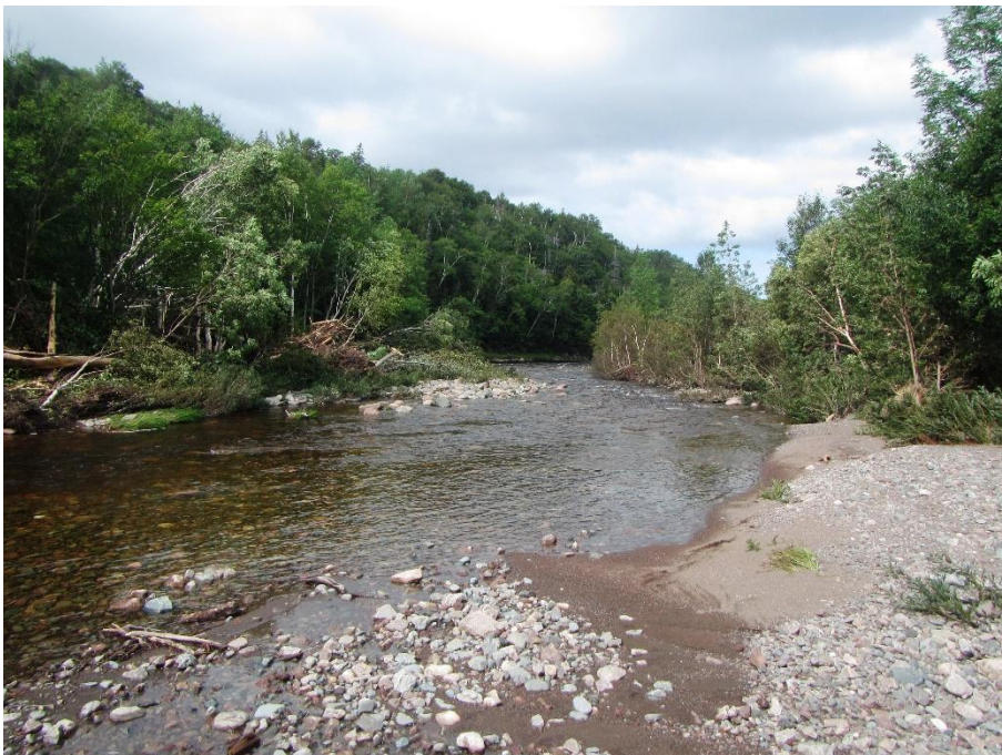
Figure 2b. View looking downstream through Robert Brook site post flood. Notice the debris and erosion on both banks
