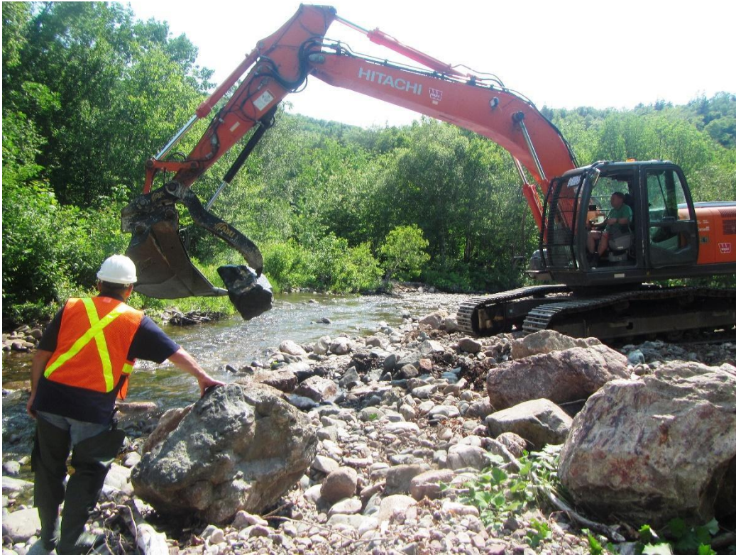
Figure 5b-2. Sill during construction in 2016
