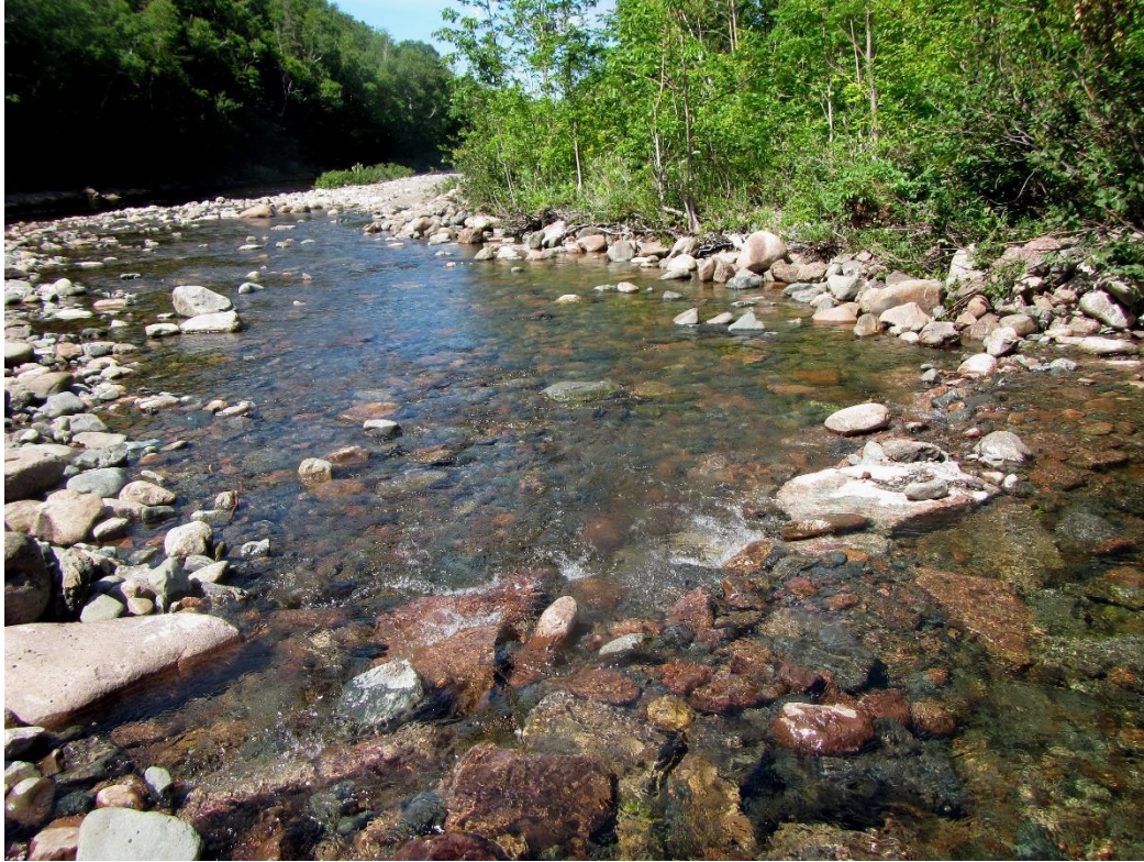
Figure 5b-3. 2016 - lower sill post installation looking downstream
