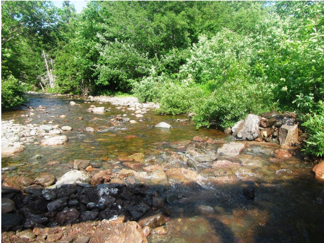
Figure 5b-4. 2016 - upper sill post installation looking upstream
