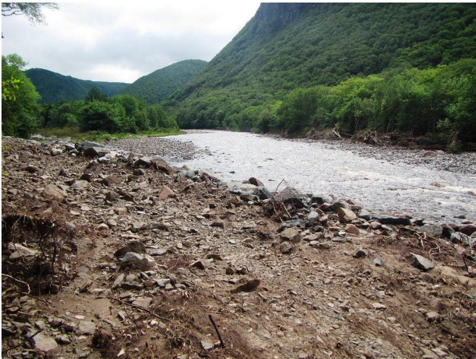
Figure 2d. View looking upstream above Fence Pool. Flood damage visible on trail and right/eastern bank
