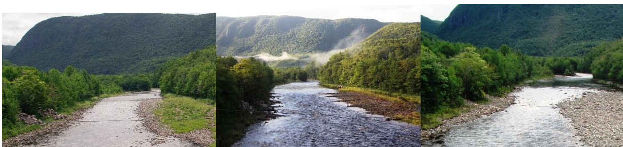
Sample project photos of the Above Cabot Trail work site in 2014 showing view looking upstream from the bridge of the channel just before work started (left), after rock retarding bars were installed (middle), and the changes to the site following major flood event in August 2015 (right).
