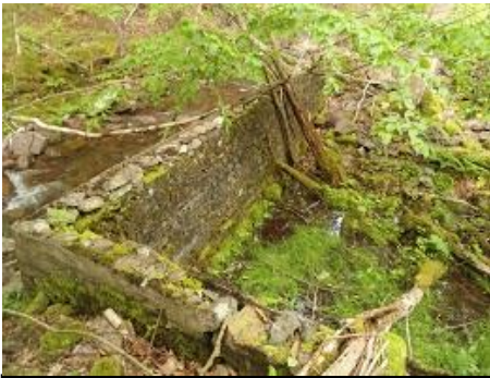
11b - Old foundation off of left bank
