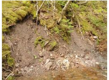
11b – Erosion, left bank
