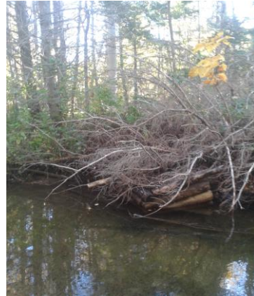
8b – Old deflector off right bank
