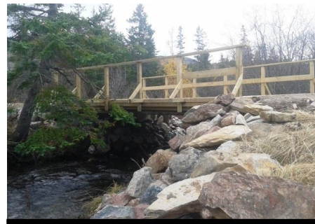
4d – Wooden trail bridge to gypsum mine (downstream view)
