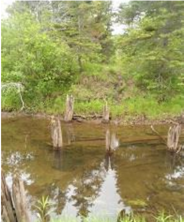
5a – Remnants of old crossing
