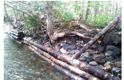
9b – Crib to help stabilize eroding left bank
