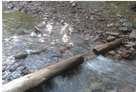
9b – Example of digger log requiring maintenance
