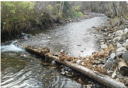
9b – Digger log and deflector requiring maintenance (DL no longer reaches right bank)
